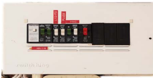
An electrical distribution board with circuit breakers
