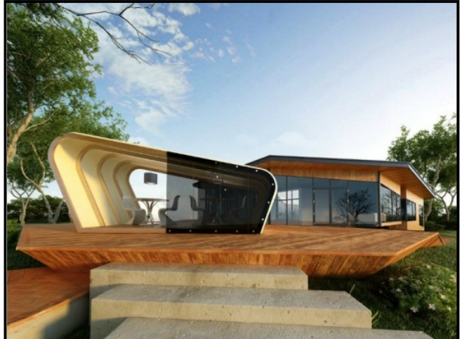
FIGURE 10b: Inflatable Pool House , AirClad Designs, opaque and solar-reflective PVC, Los Angeles (USA), 2012.
