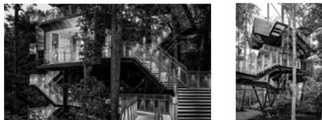
**The Sustainability Tree house** is 126 feet tall and 4000 square feet structure.  The tree house is constructed from Corten steel frame and luminous wooden box platforms.  It is designed with a plethora of green building systems such as photovoltaic panels,  wind turbines, large cistern and a water cleansing system.
