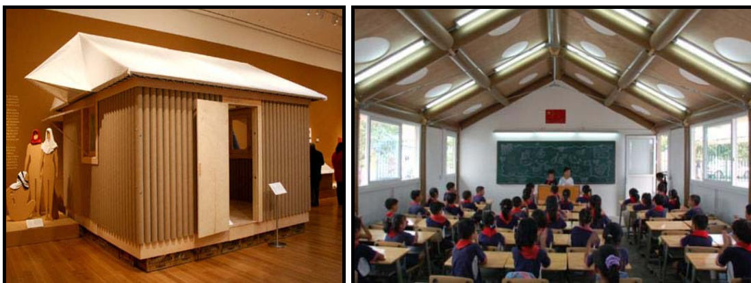
Left: a shelter constructed from paper and cardboard. Right: a paper-tube school in China.
