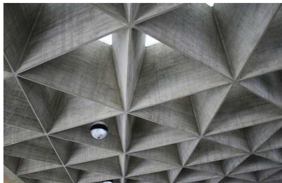
A roof in an airport where the structure is made stronger by using triangle shapes which are very strong.
