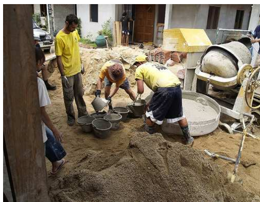
Mixing cement using a mixer.
