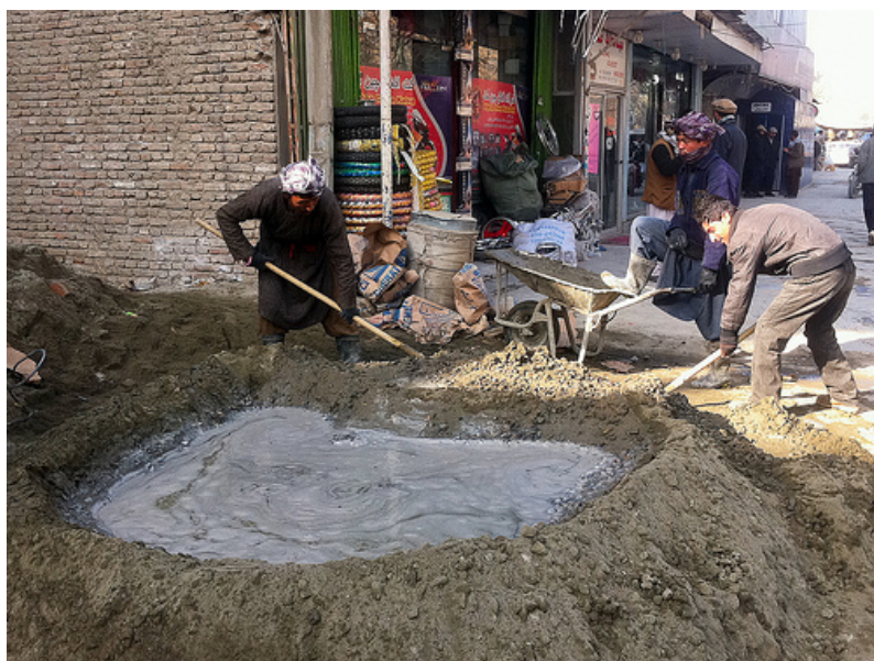
Mixing cement using spades.
