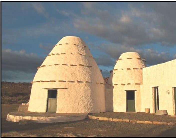
FIGURE 8a: Whitewashed corbelled houses , stone, mud and clay, Stuurmansfontein Farm, Karoo, 19 th Century (built by nomadic farmers)
