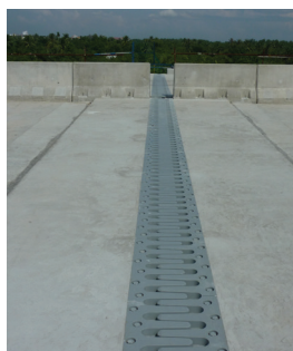
Figure 5.33 The expansion joint in a bridge.
