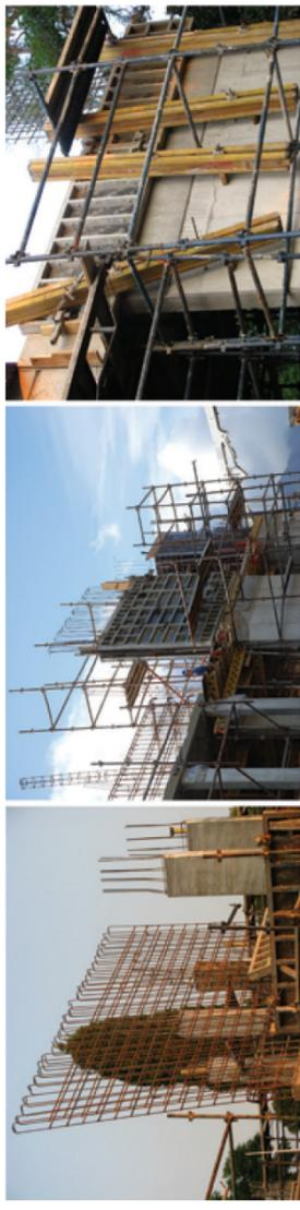
Figure 20: Steel reinforcement is placed inside a concrete wall of a big building.
