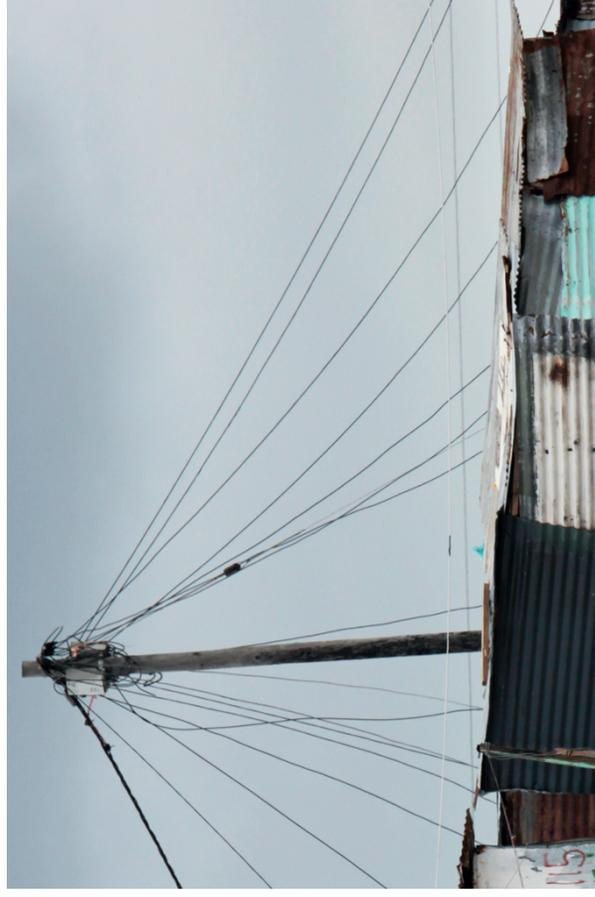
Figure 5: An informal community with an electrical supply. Notice the control boxes at the top of the poles. They control how much electricity each household uses and have a built-in safety mechanism for when there is a short circuit.
