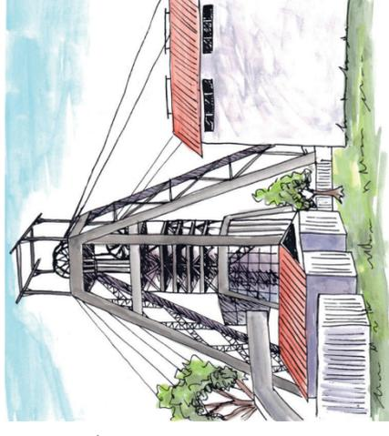
Figure 4: The headgear of an underground mine. The shaft goes straight down into the ground under the wheels of the headgear, sometimes kilometres deep.
