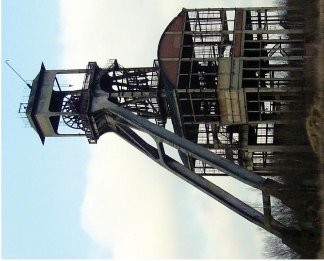
Figure 1: This is the tower above an old mine shaft. A cable winds around “sheave” wheels on the “headgear” at the top. These cables are attached to a lift that transports miners, machines and ore into and out of the mine.
