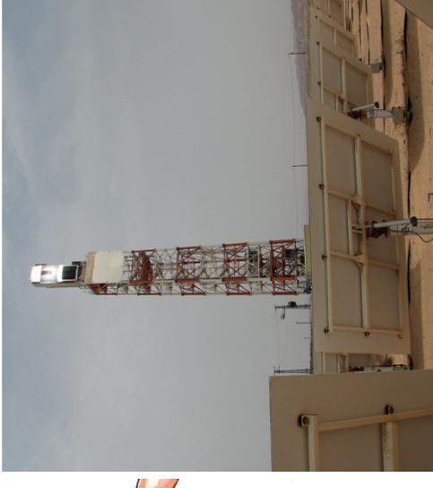
Figure 9: Many mirrors can be used to reflect a lot of sunlight onto a small tin can, to heat water in the can. Figure 10: Thousands of mirrors at a solar thermal power station all reflect sunlight onto a tank on top of a tower. That is why the tank is shining so brightly.
