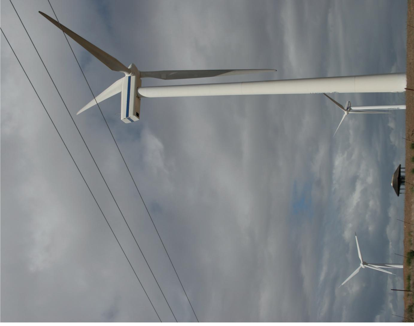
Figure 8: A wind turbine generates electricity by using the force of the blowing wind. The blades of the turbine are made of a synthetic material called “epoxy resin,” that is combined with fibres. This makes the blades very strong, but at the same time very light. Also, it is possible to make this material into a special shape.
