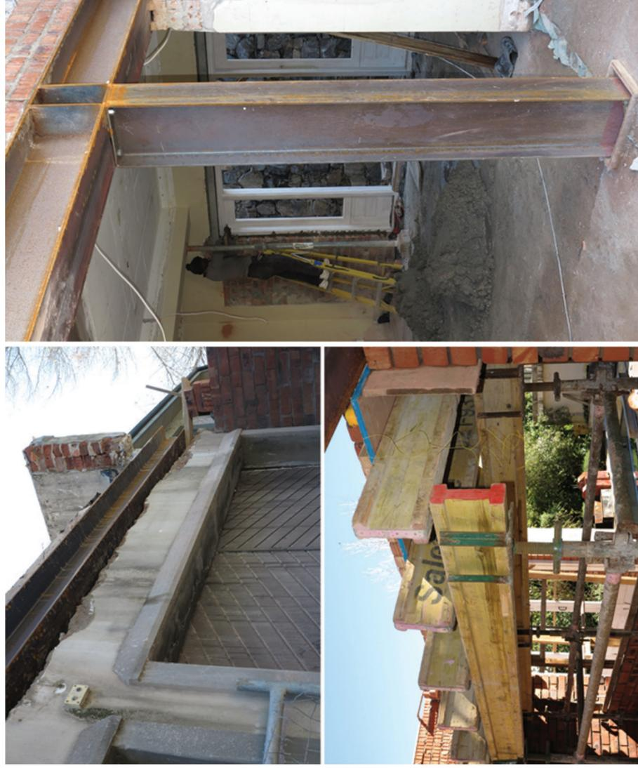
Figure 25: Steel I-beams are often used in buildings. Wood I-beams are often used during the construction of a building, but are removed once the building can support its own weight.
