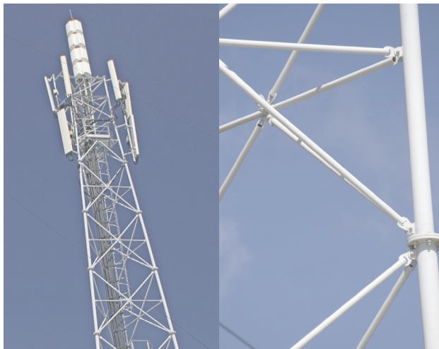
Figure 3.20a The steel columns of this cell phone tower are heavier than all the other members
