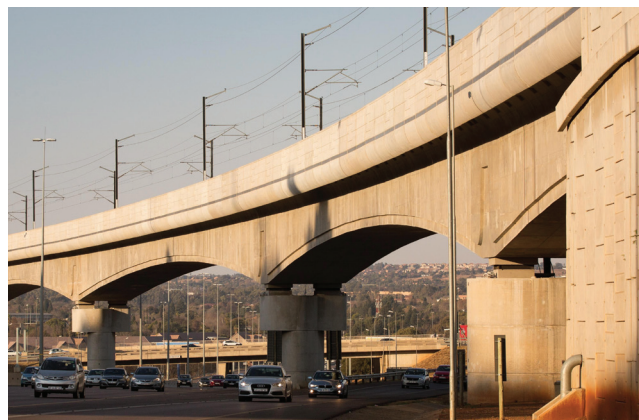
Figure 5.9d There is a bearing between each of these supporting columns and the bridge structure above.
