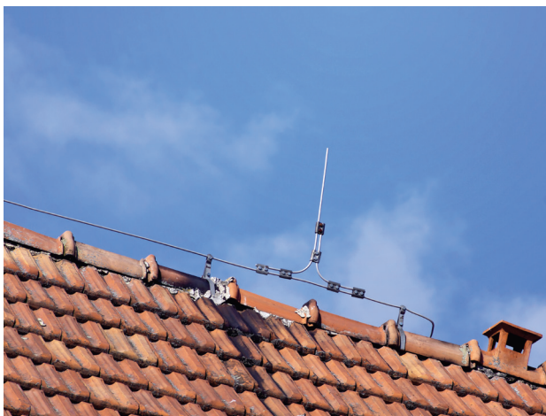
Lightning rod wire on a roof of clay tiles
