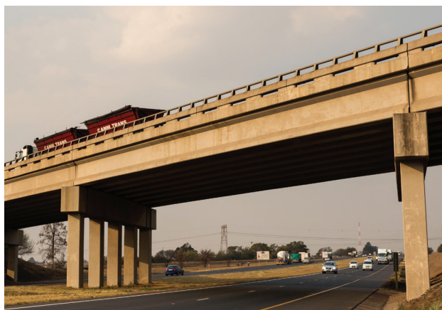
Figure 5.10a Simply supported beams in a bridge
