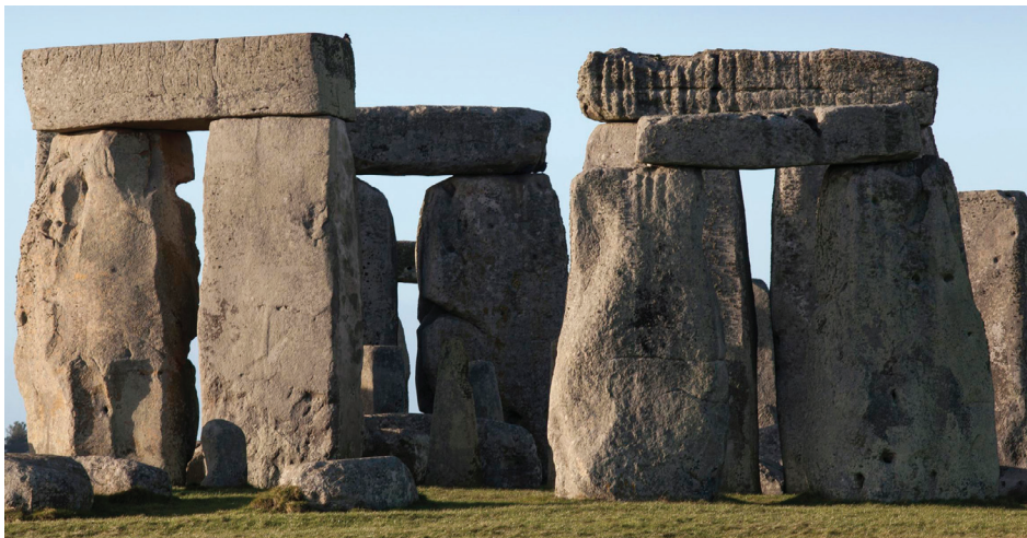
Figure 5.8 Ancient beams were usually simply supported.
