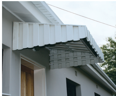
Figure 5.38 Three different cantilevers: to support shade cloth; to support a canopy over a door; as part of a precast bridge section
