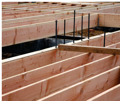
Figure 3.24a Wooden floor joists
