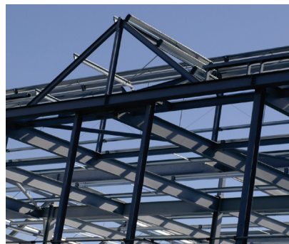
Figure 3.24c Steel beams in a steel-framed building
