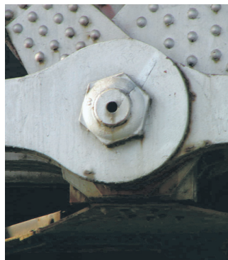
Figure 5.9a A pinned joint
