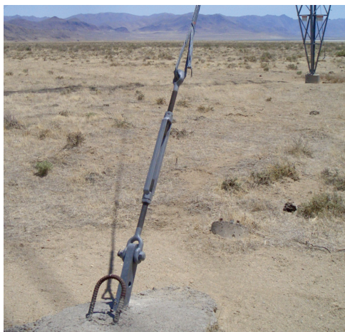
Figure 3.17a Cable stabilising a tower
