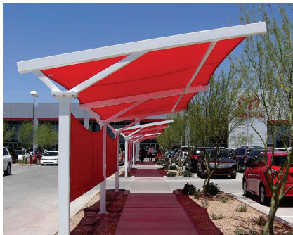
Figure 5.38 Three different cantilevers: to support shade cloth; to support a canopy over a door; as part of a precast bridge section
