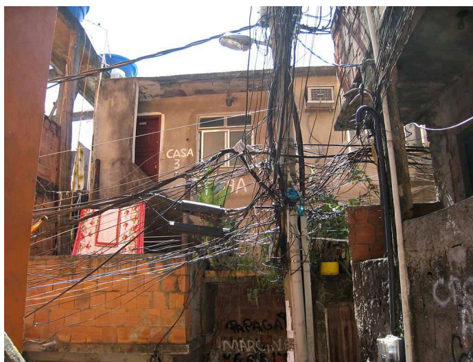
Look at this mess of illegal electrical connections. 4
