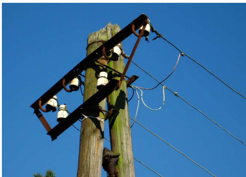
In this photo, the wooden poles and white ceramic caps are electrical insulators.
