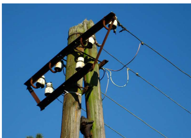
The wooden poles and white ceramic caps are electrical insulators.
