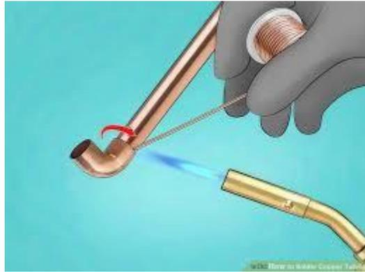
Solder continuously added to joint.
