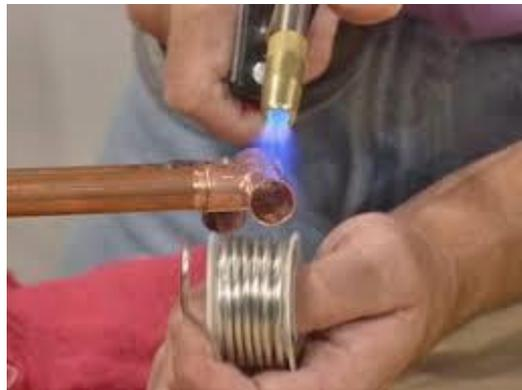
Add solder and applying heat at the correct temperature.
