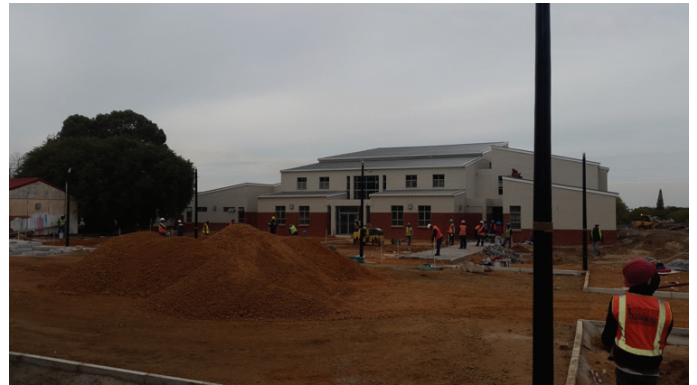
Work in progress in Atlantis
