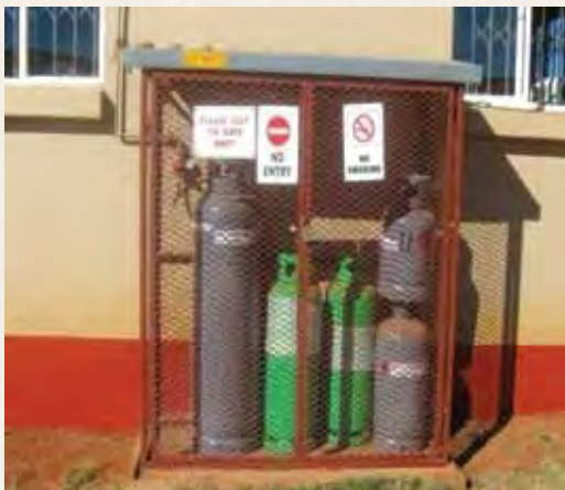
Store gas cylinders in lockable steel cages with clear safety signage
